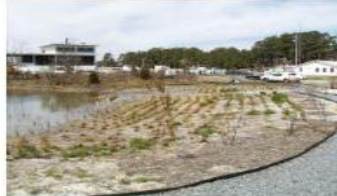
A degraded upland and wetland area was excavated and graded to create a planted marsh at VIMS. Note the gradual slopes and rapid plant growth after the first growing season. Photos by K. Duhring
