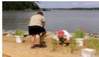
The planting process includes pre-drilling holes then inserting a plug into each hole. It's very important to pack the soil around each plug to remove air pockets. A small quantity of slow-release fertilizer can be placed in the hole under each plug, but this step is not essential for successful plant growth. Photo by K. Duhring
